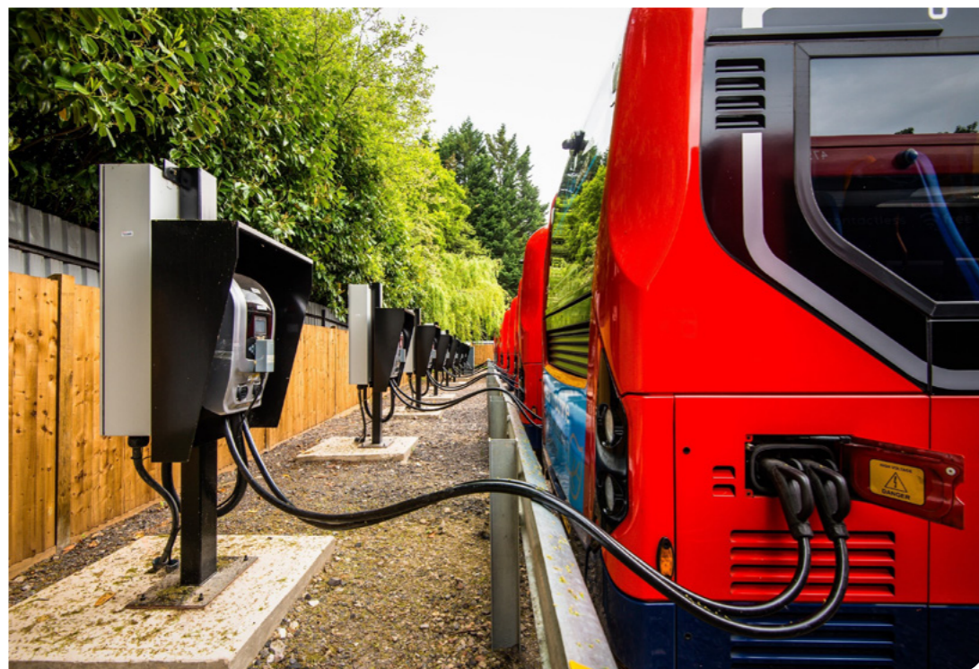
Figure 6: Dual AC Type 2 charging system plug and vehicle interface providing 86kW of charge through two 43kW dual chargers.
